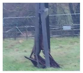
Central trestle leg of the Headstocks, highlighting significant deterioration. This was picked up during a routine structural condition check by employees.
